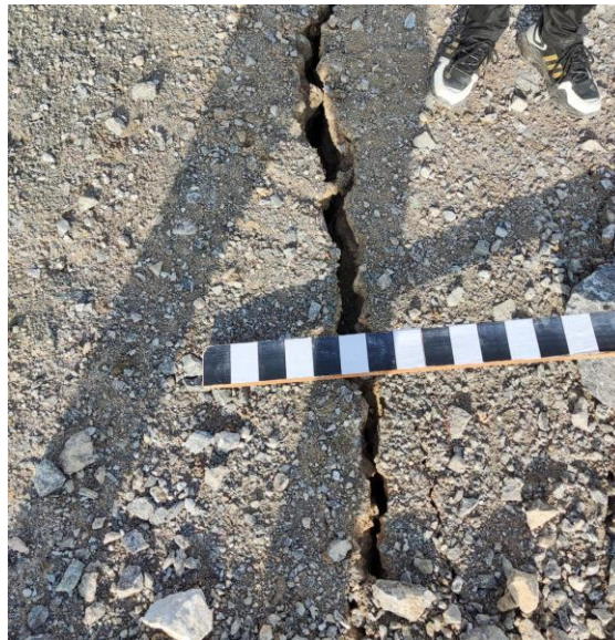
Fig. 1. The separation of the array after drilling and blasting.
